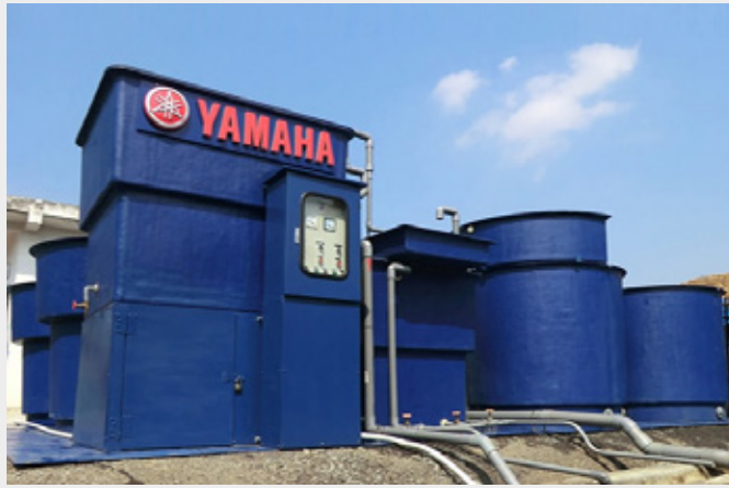
Yamaha Clean Water Supply System produces drinking water from surface run off
