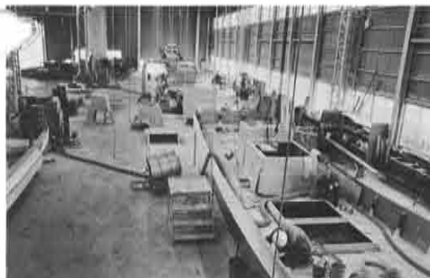
Hull-deck assembly
