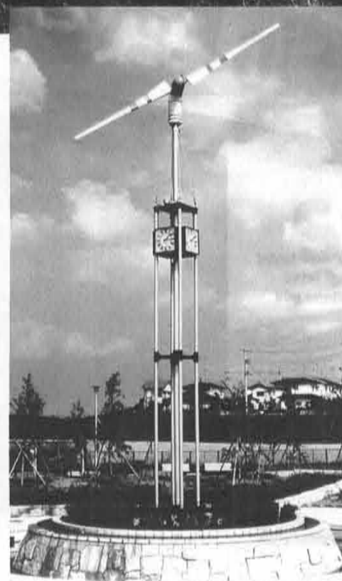
An existing monument-type Yamaha wind-turbine generator.
