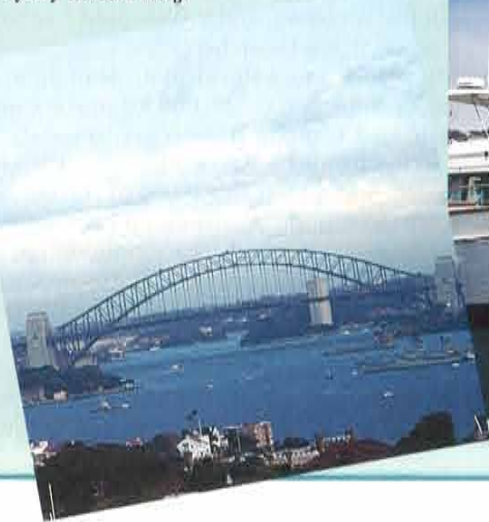
Sydney Harbour Bridge
