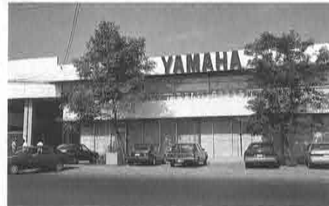
YMMEX new office building.
