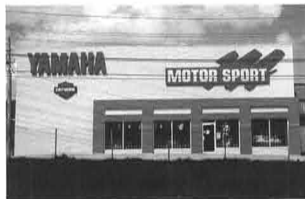
The new Motor Sport office and showroom facility
