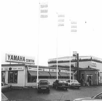
The Yamaha Center building is completely restored and gives a positive impression
